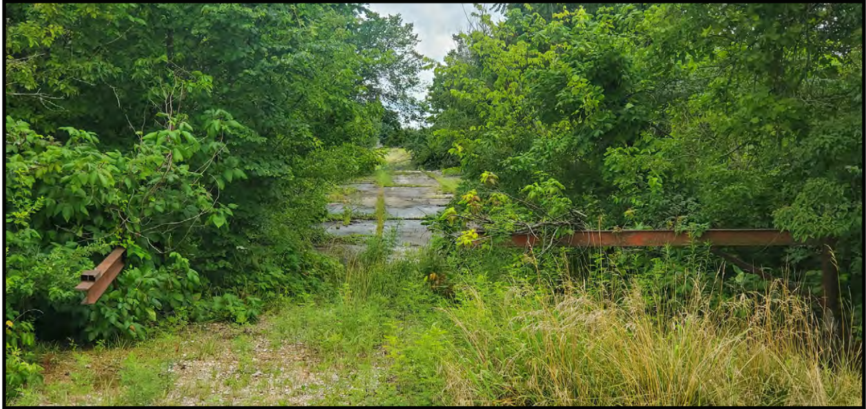
Figure 10. Overview of the eastern portion of the Lawrence Dragway. Note, this segment of the Dragway was not in the Project area. View is to the west. Photo by Shannon R. Ryan, 7/4/24.
