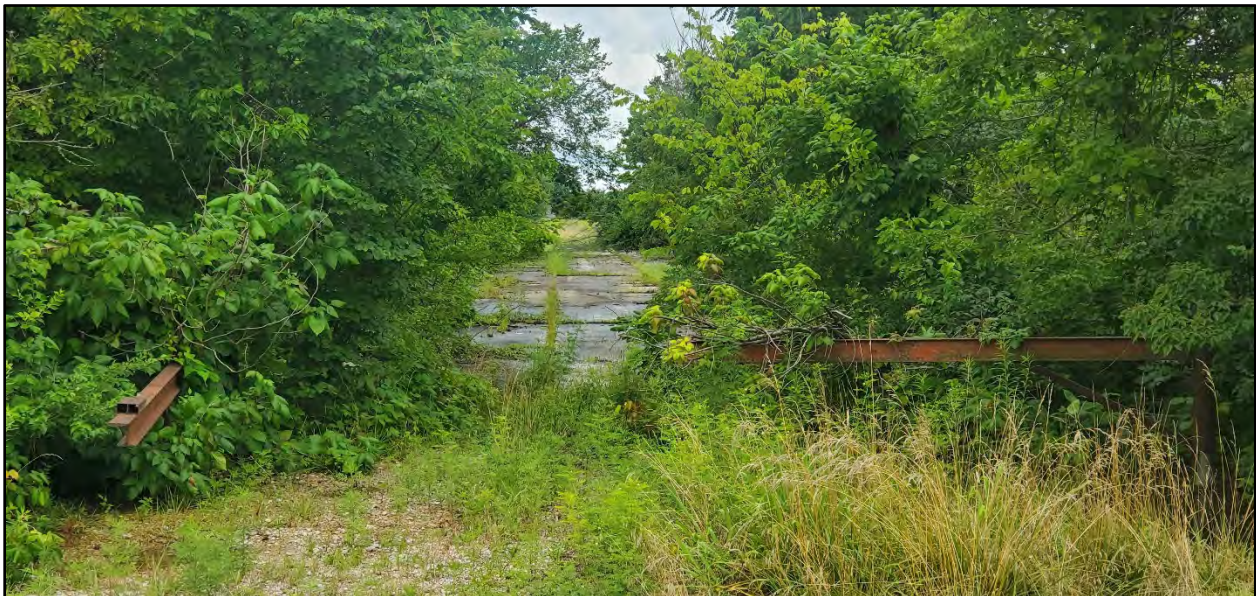
Figure 7. Overview of the eastern portion of the Lawrence Dragway as it appeared in July 2024. Note, this segment of the Dragway was not in the area surveyed. View is to the west.
