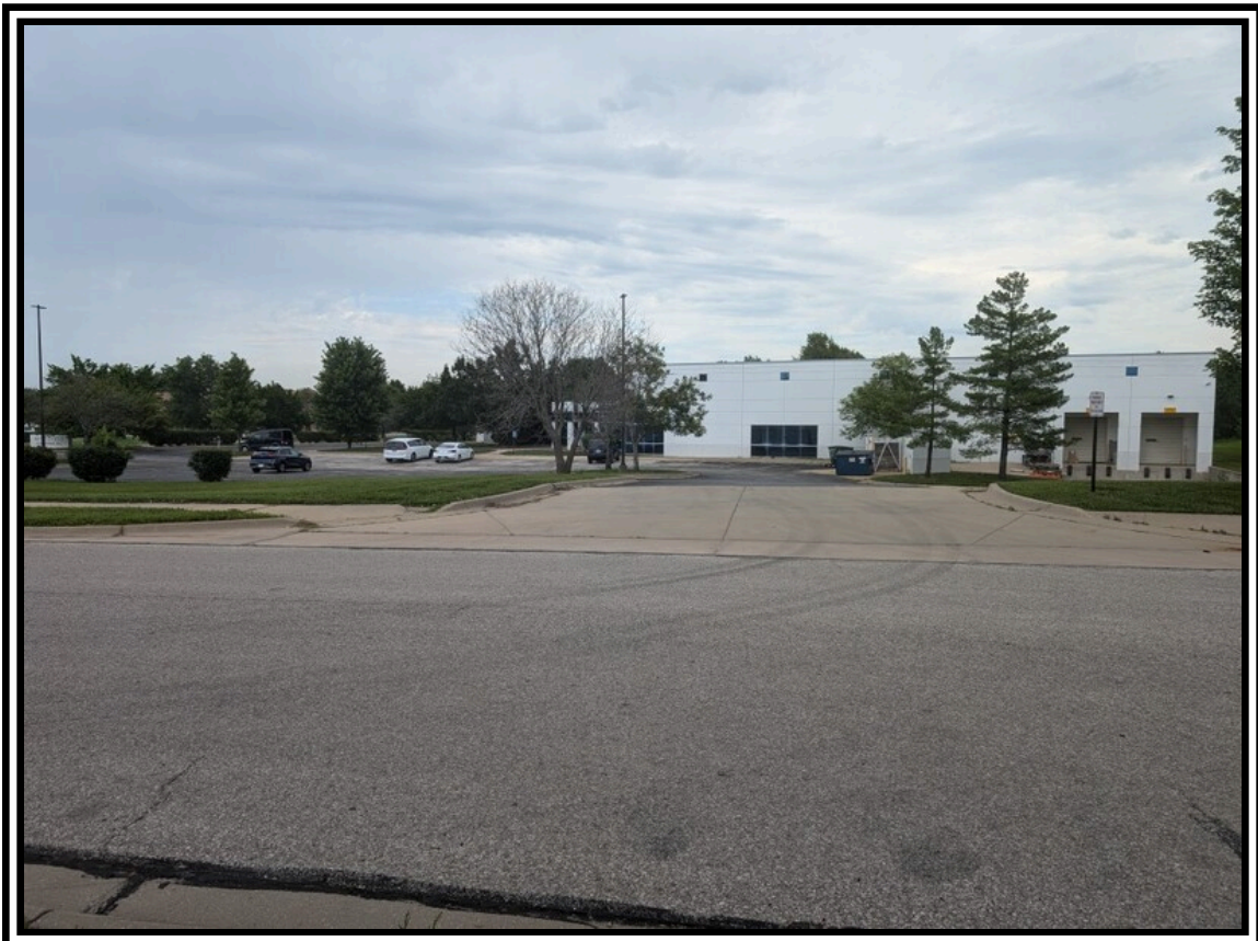
18: Adjoining Commercial Building, Northeast
