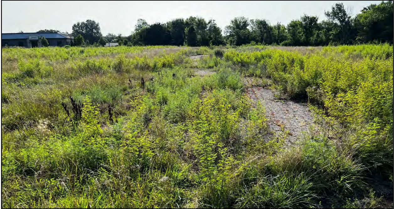
Figure 6. Overview of the Lawrence Dragway (14DO262, Feature 1) in an overgrown lot; view is to the east.
