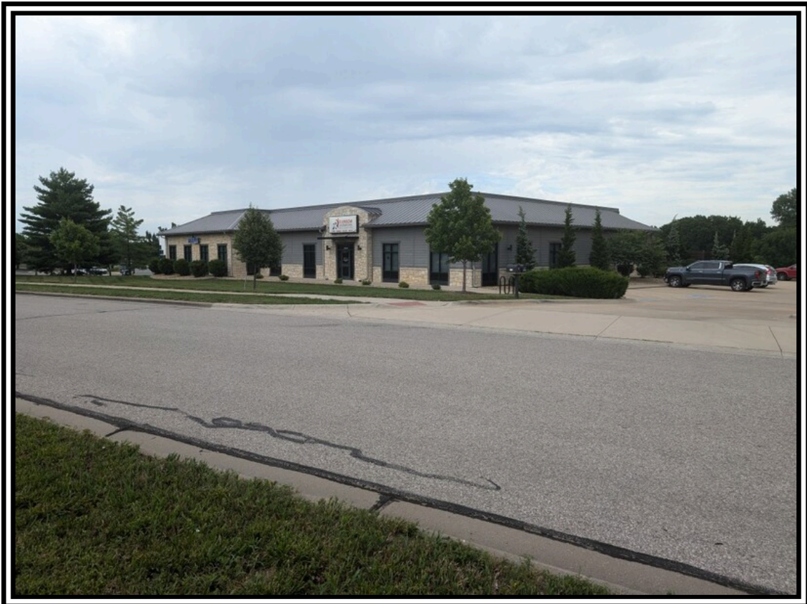
19: Adjoining Commercial Building, East
